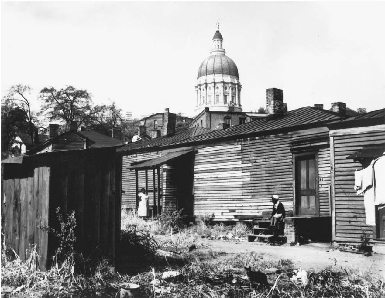
These dilapidated buildings stood on the Georgia State Capitol Homes site in Atlanta, Georgia, before the U.S. Housing Authority demolished them and began a construction project on the site during the late 1930s. FRANKLIN DELANO ROOSEVELT LIBRARY
