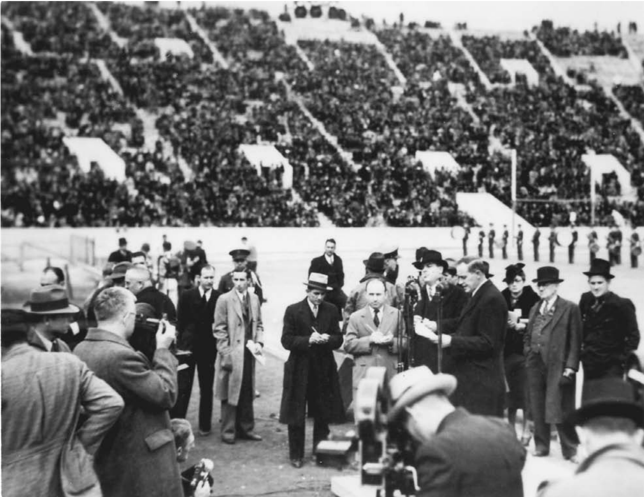
Harry Hopkins (right, at microphone) speaks at the dedication of the Louisiana State University Stadium, a WPA construction project, in November 1936. FRANKLIN DELANO ROOSEVELT LIBRARY
