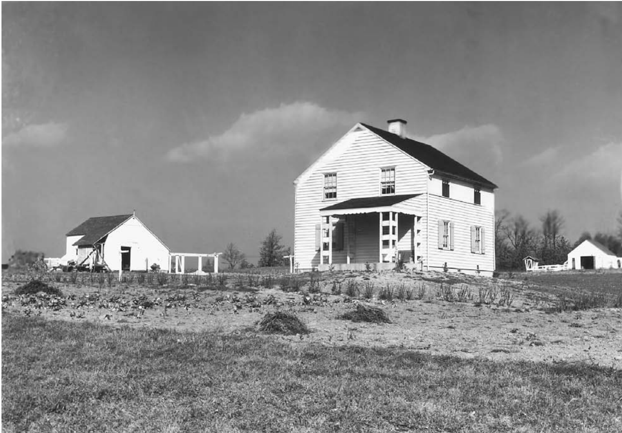
This homestead in West Virginia was built during the mid-1930s as part of the Farm Security Administration's Arthurdale project. LIBRARY OF CONGRESS, PRINTS & PHOTOGRAPHS DIVISION, FSA/OWI COLLECTION
